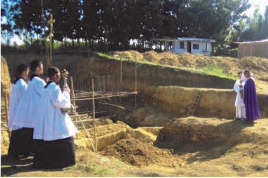
Fr. Cacho blesses the foundations and consecrates the pillars of the new church.
