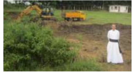
... then Fr. Baudot, the great Bursar from HQ, discovers the project, ...
