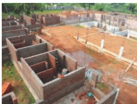
The huge building project is half complete.
